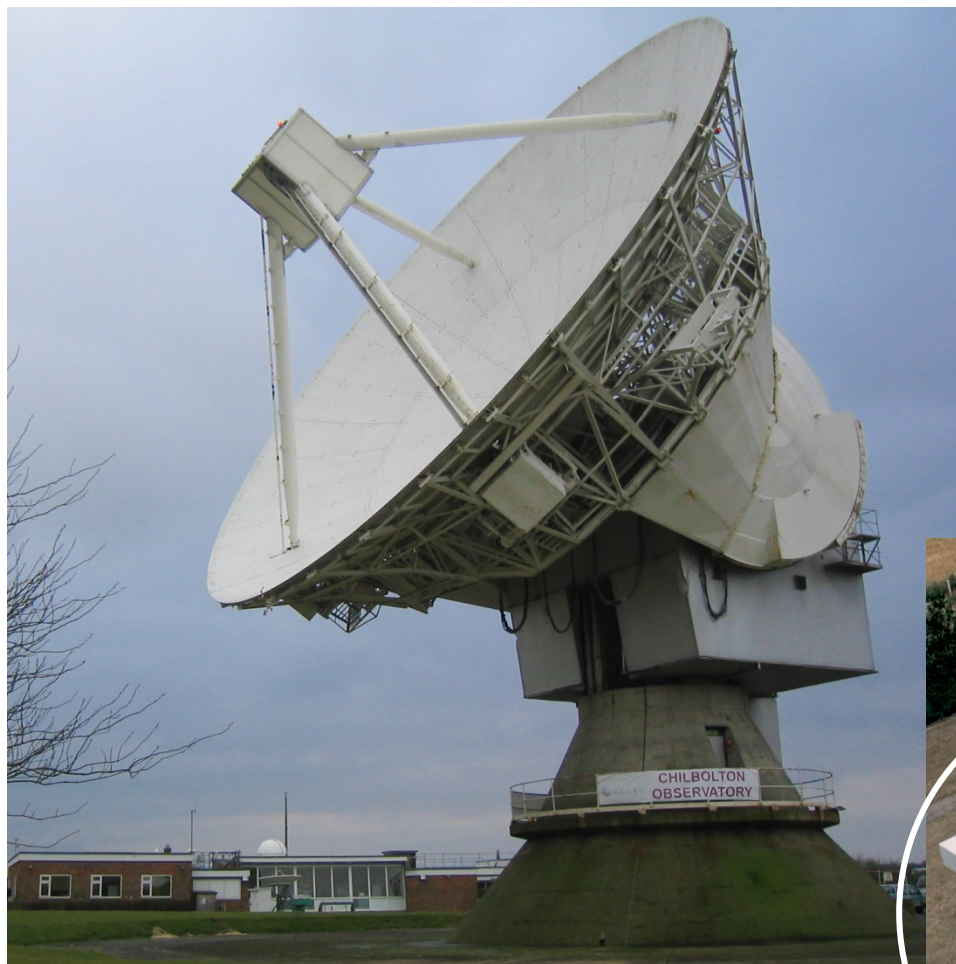
25 m antenna of the S-band weather radar at Chilbolton, UK
